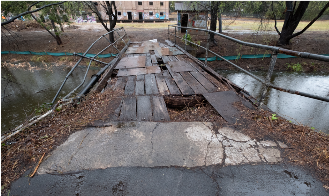
Figure 40 : Road bridge over creek opposite Malthouse 3, a weir is located under the bridge. Note its deteriorated condition. It is to be reinstated as part of the works. Paul Davies 2019.
