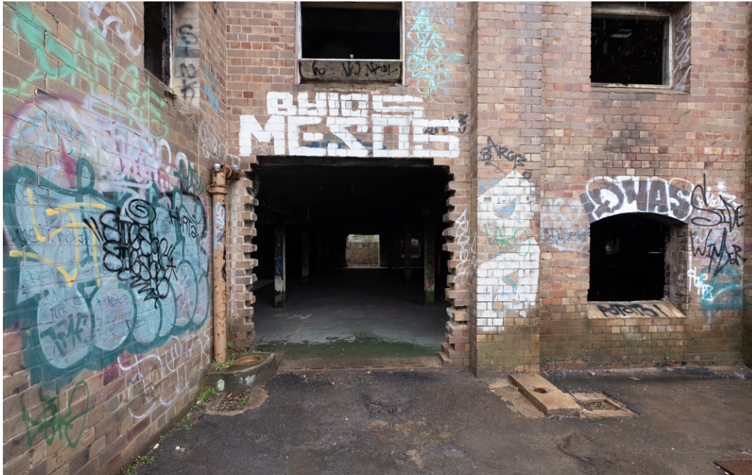
Figure 38 : Malthouse 2, formerly a window, the wall has been removed to provide for access. This will form a new major entry into the building with access to the upper floors. Note that windows do not have any remaining joinery. Paul Davies 2019.
