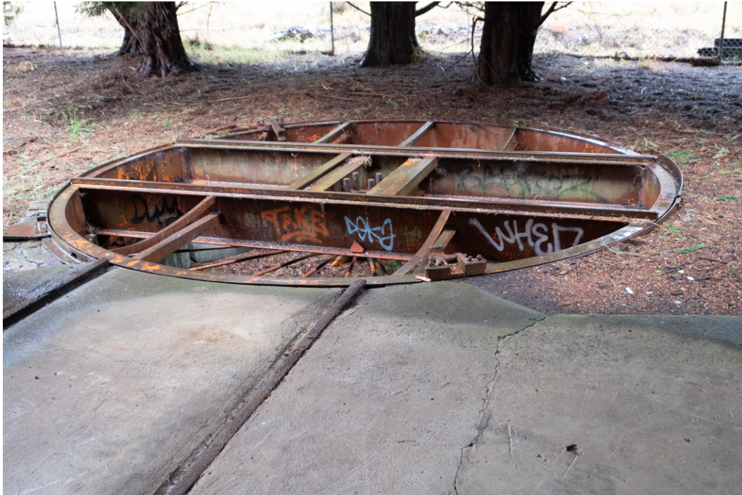
Figure 42 : Rail turntable that remains in situ with some remnant tracks. Used to move trucks between the Malthouse 1 grain stores, across the bridge and to and from Malthouse 3. It is retained and conserved. Paul Davies 2019.
