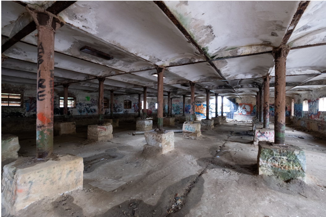
Figure 34 : Basement level of Malthouse 1 showing the steel structure and coffered concrete soffit to the floor above. The concrete floor is now exposed to the weather as the upper floors were destroyed by fire. This area has been excavated as part of works in the 1980 period. Paul Davies 2019.
