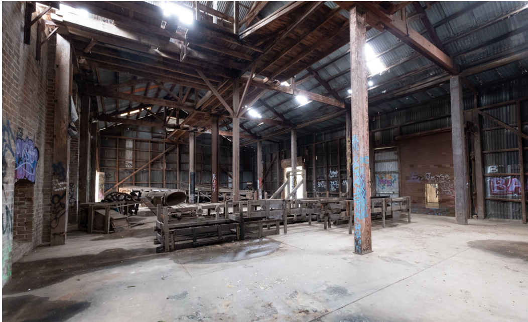
Figure 36 : Maltstore 1b with the Malthouse on the left. A combination of steel and timber framing and clad with corrugated iron. Some remnant machinery is stored in the building. Paul Davies 2019.
