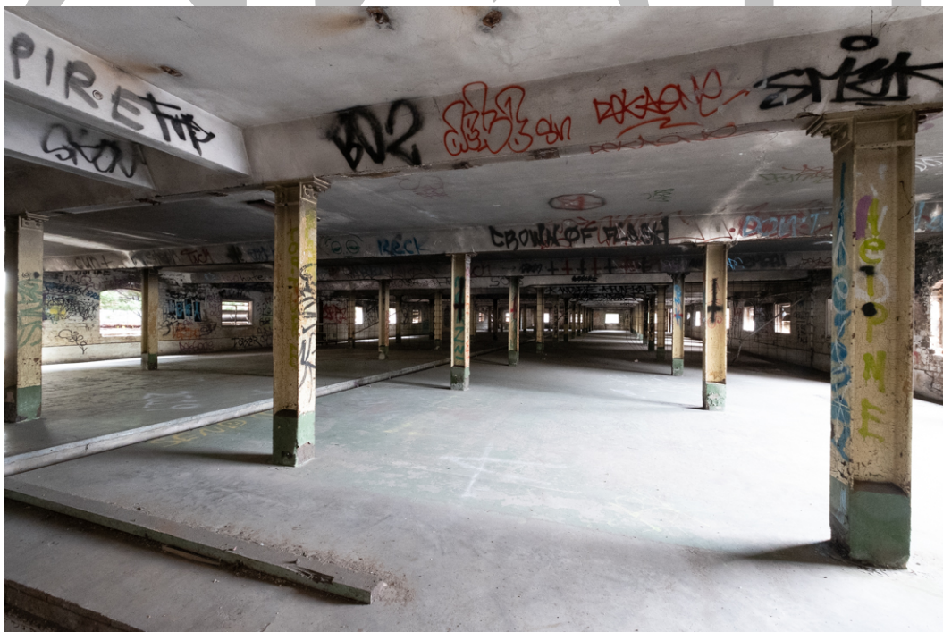
Figure 35 :Ground level of Malthouse 2 with machinery trench to the left. The dense layout of steel columns supported floors above,note the low head height in relation to other floors. This area will become back of house and the new entry to the upper level. A section of floor is to be removed to allow for lifting. Paul Davies 2019.
