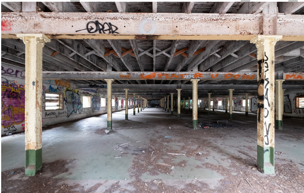
Figure 37 : First floor of Malthouse 2, a drying floor with relatively low headroom and a heavy steel structure. Paul Davies 2019.
