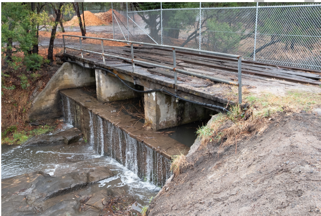
Figure 41 : Road and rail bridge near Malthouse 1 with rail tracks remaining and concrete weir. It has been reinstated as emergency works. Paul Davies 2019.
