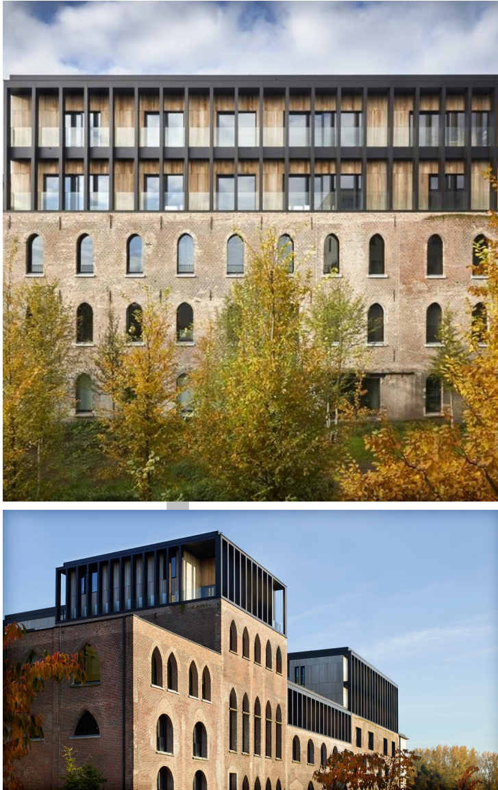
Figure 15: Distillery Antwerp (former Maltings complex) Vervoordt 2017 Retention of the façade brickwork and a well-modulated vertical addition.
